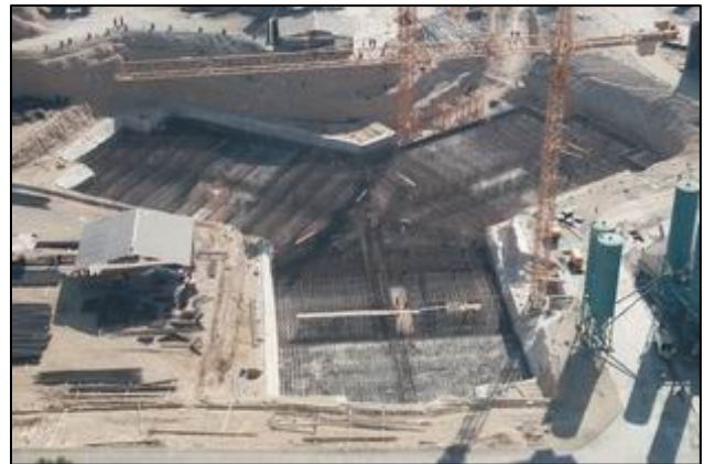
Figure 2. The view of the structural foundation.
