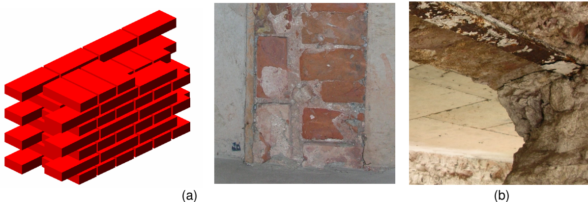
Figure 8. a) Brick arrangement of the masonry walls, b) the steel tie.
