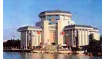
Figure 8. RC frame-shear 13 stories museum with story isolation.
