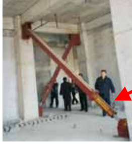
Figure 18. Building bracing with oil Damper.
