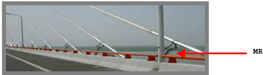
Figure 28. MR is used in Ton-Tin Lake Bridge in China.
