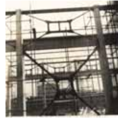
Figure 15. The 1 st structure with damper in China.
