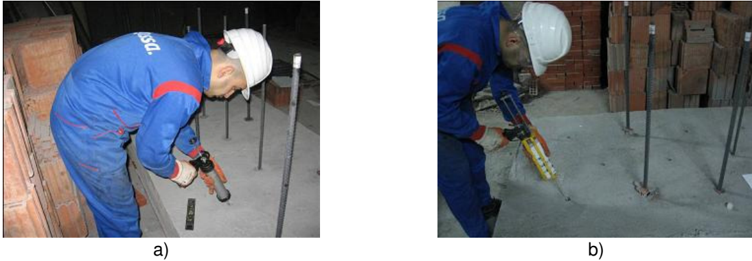
Figure 3. Filling the holes with a) M1 and b) M2 adhesives, respectively.
