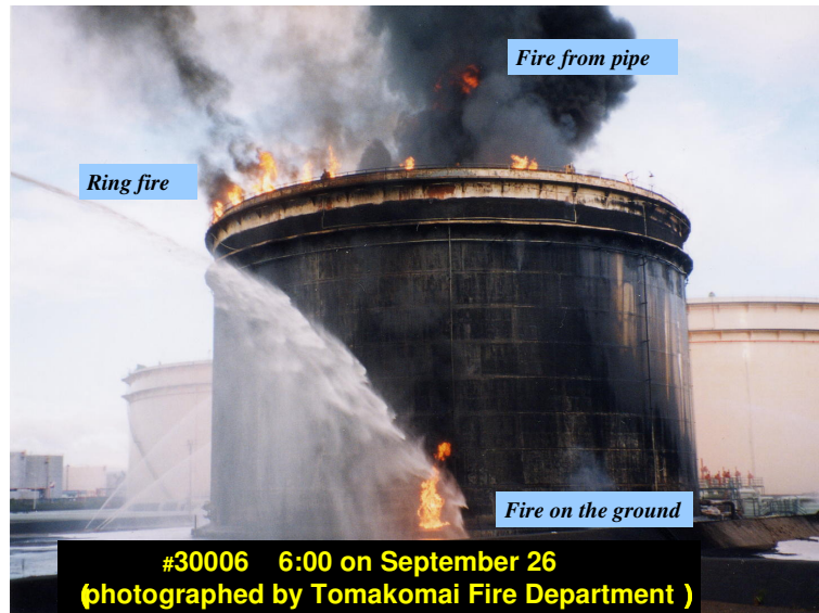
Figure 5. Tank fire just after the earthquake (photo by Tomakomai Fire Service).
