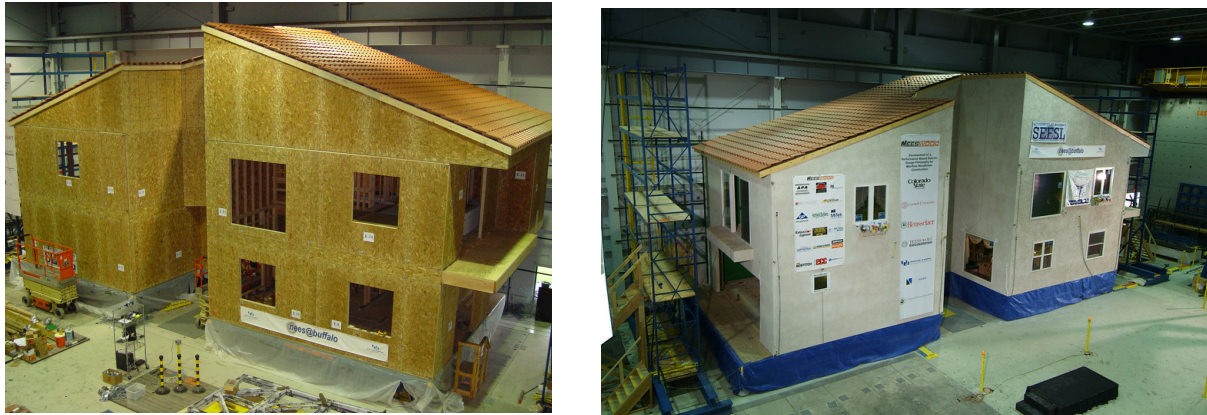
Figure 3. Benchmark Test Structure During Phase 1 (OSB Only) and Phase 5 (All finishes).
