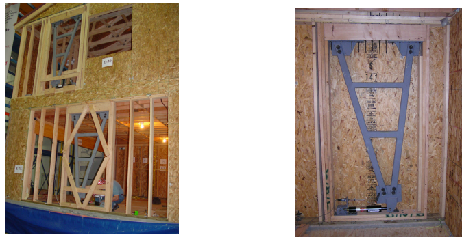
Figure 5. Prefabricated Damper Walls - Phase 2.
