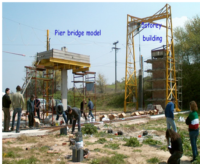
Figure 1. Overview of the Test Site facilities.
