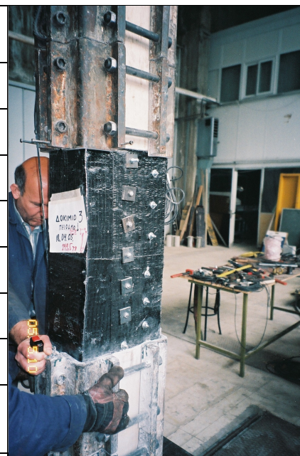
Figure 5. Confining steel brackets and partial CFRP confinement at the mid-part.
