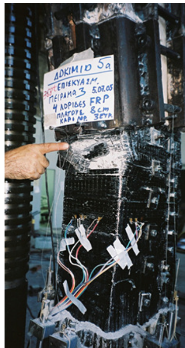
Figure 11b. Failure of the CFRP layers of the mid-part.
