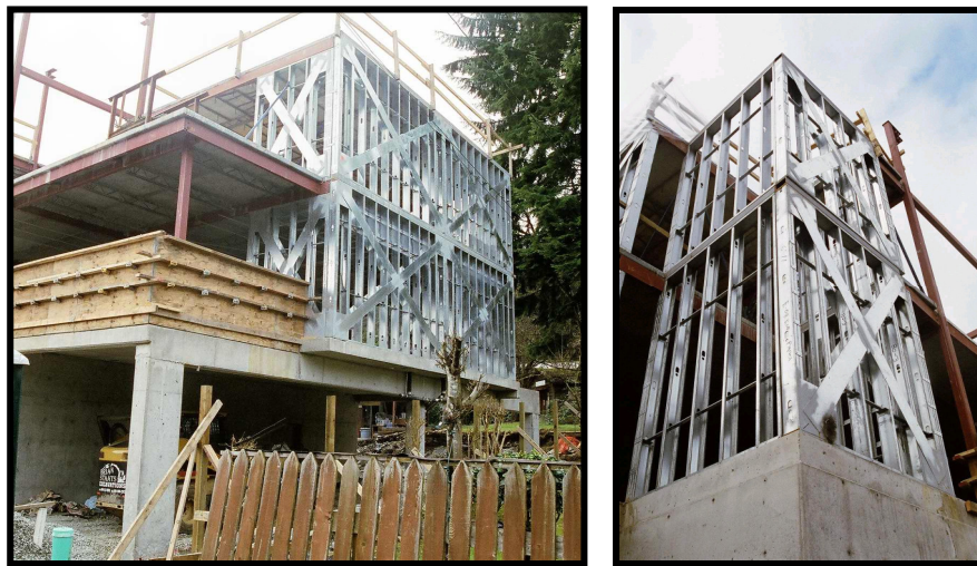
Figure 1. Cold-formed steel strap braced walls under construction.
