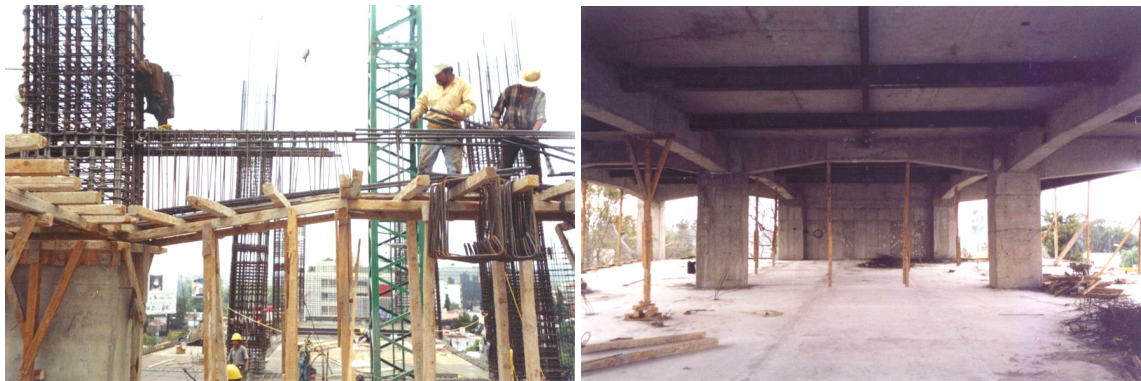
Figure 1. RC buildings with haunched beams recently constructed in Mexico City.
