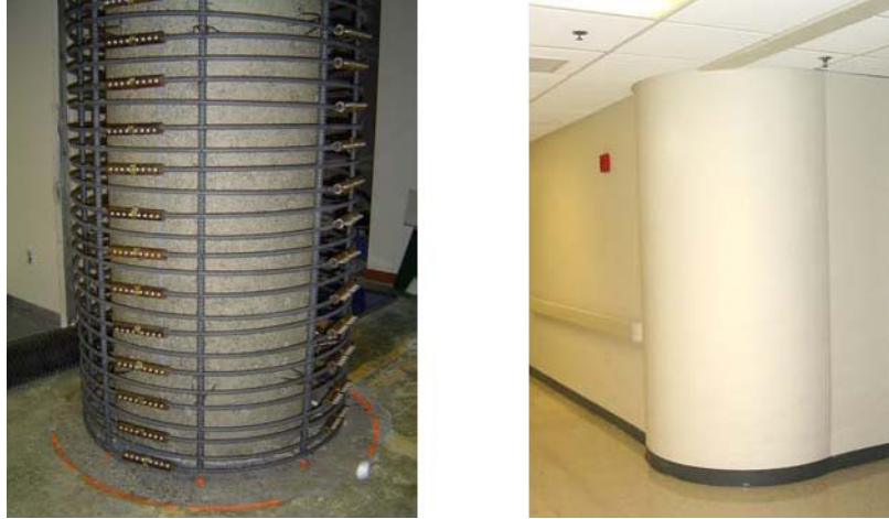
Figure 7. Concrete Column Enlargement Before and After.
