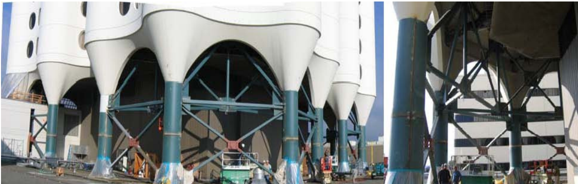
Figure 9. Completed Damper Installation.
