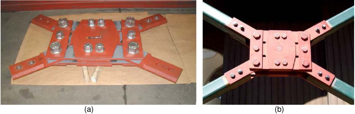
Figure 4. (a) Prototype Friction Damper and (b) Installed Friction Damper.
