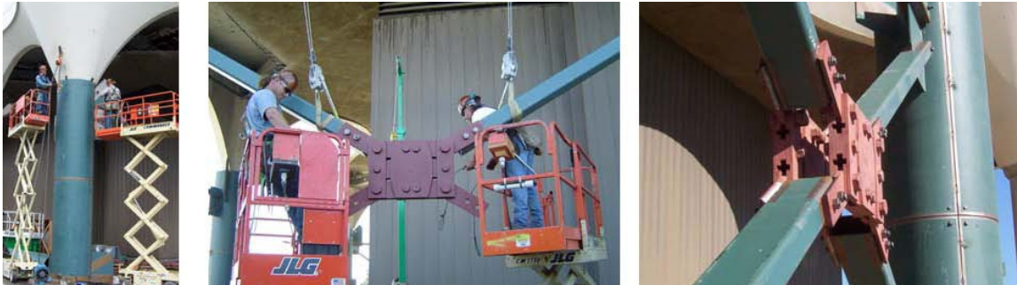
Figure 8. Steel Jacket and Damper Installation.
