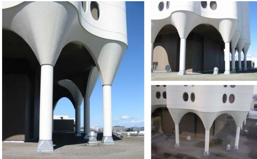
Figure 2. Existing Building Soft-Story.
