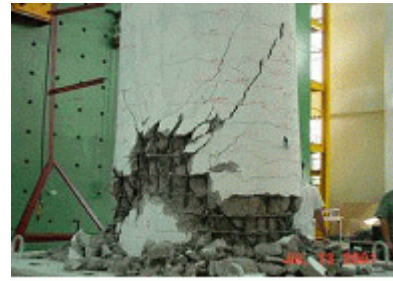
Figure 6. Failure of MD-HT6-N-L2.
