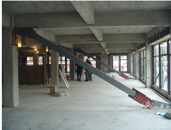
Figure 9 Retrofitting of existing structure with Pall friction dampers
