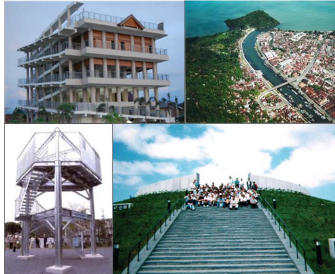
Figure 2. Examples of tsunami evacuation structures. (Top left) Tsunami evacuation building in Banda Aceh, built after the 2004 tsunami. This building’s secondary purpose is to serve as a community center. (Bottom Left) Pre-fabricated structure in Japan with the sole purpose of serving as an evacuation site during a tsunami. (Top right) Aerial photo of a bridge in Padang that provides access to high ground from the city center. (Bottom Right) A soil berm in Japan that provides refuge during tsunamis. Image sources: ATC-64.
