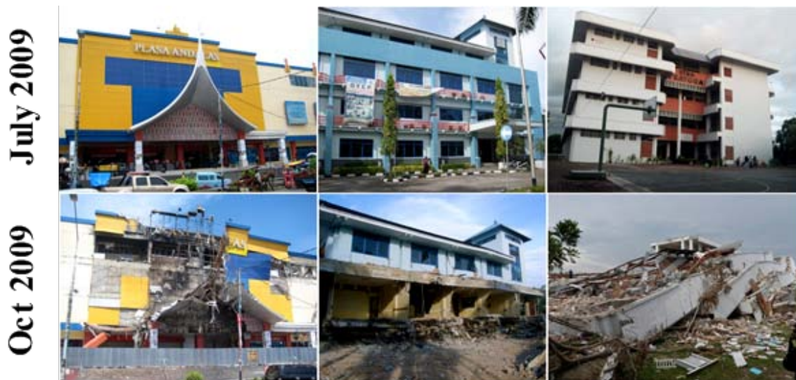
Figure 4. Before and after photos of buildings that had been recommended as evacuation sites. From left to right: Four story mall, partial collapse on the 4 th floor and fire; 4-story language school, collapse of first 2 stories; 4-story junior college, complete collapse. Image source: EERI.
