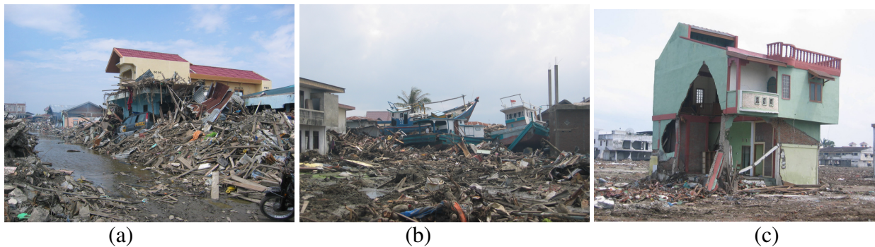
Figure 3. Tsunami damage in Banda Aceh, Indonesia, 2004 Indian Ocean Tsunami
