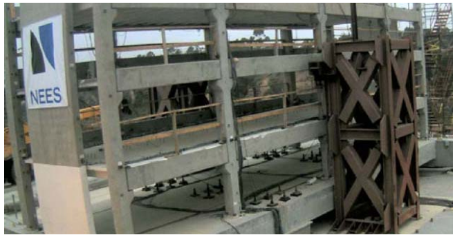
Figure 2. Testing a three-story, half-scale precast concrete parking garage on the NEES shake table at University of California San Diego.
