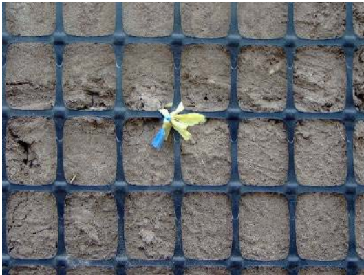
a) Geomesh tied to adobe wall (A. Rubiños)
