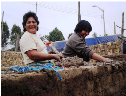
a) People placing mortar mud
