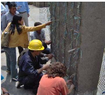
a) Geomesh placement training wall
