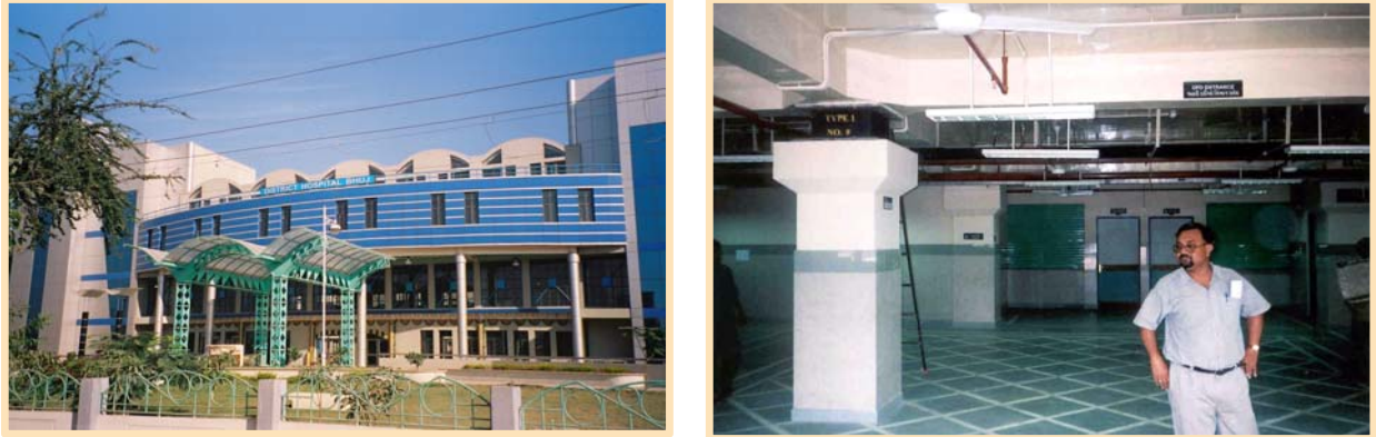
Figure 13. Bhju District Hospital (RSL 2009)
