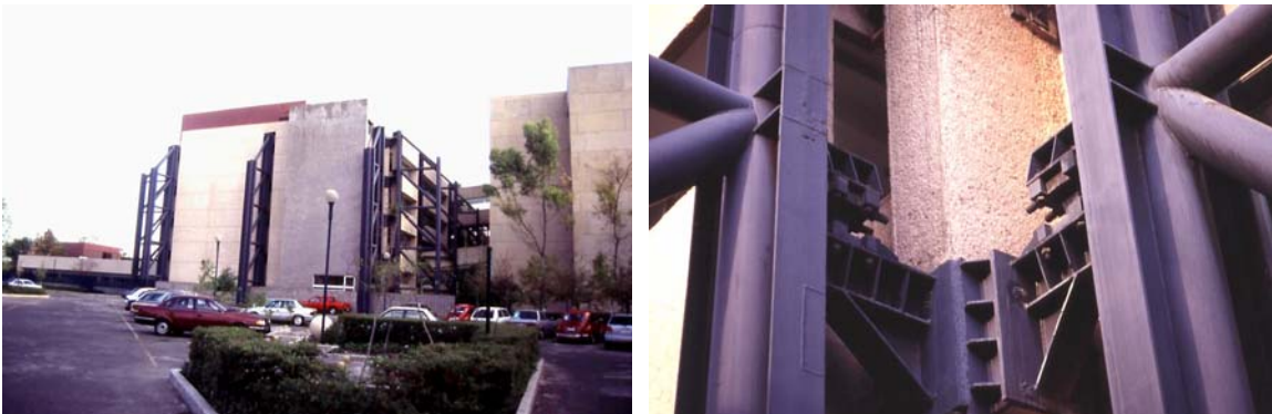
Figure 5. Retrofit of IMSS Cardiology Hospital with ADAS devices
