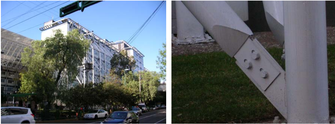
Figure 6. Retrofit of November 20 th Hospital Complex with slotted-bolted-connections (SBC)
