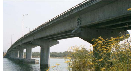
Figure 1. Humboldt Bay bridge.
