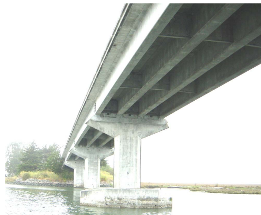
Figure 2. Bridge (close-up view).
