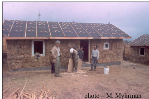
< Fig.1. Load-bearing house. Mongolia
