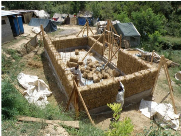
Figures 4 and 5. A PAKSBAB house under construction, and completed (2009). (photos D.Donovan)
