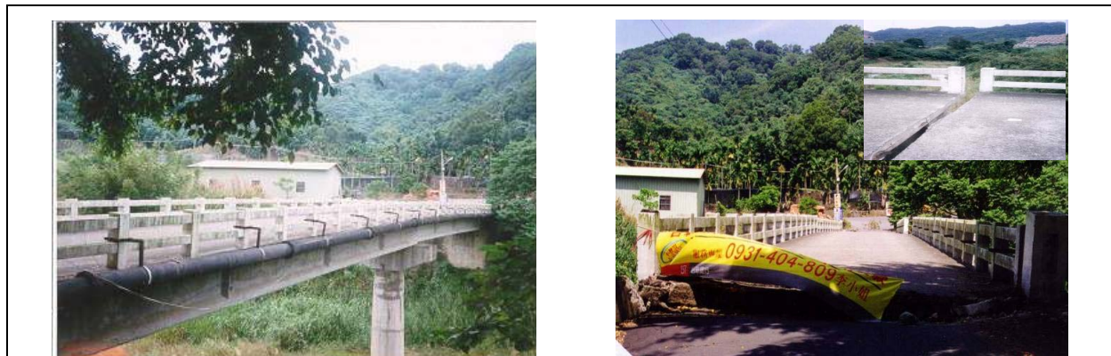
Figure 1. Sliding/Friction Mechanism of bearings in Kuan- Lung bridge (439 Gal recorded PGA) during the Chi- Chi Earthquake.
