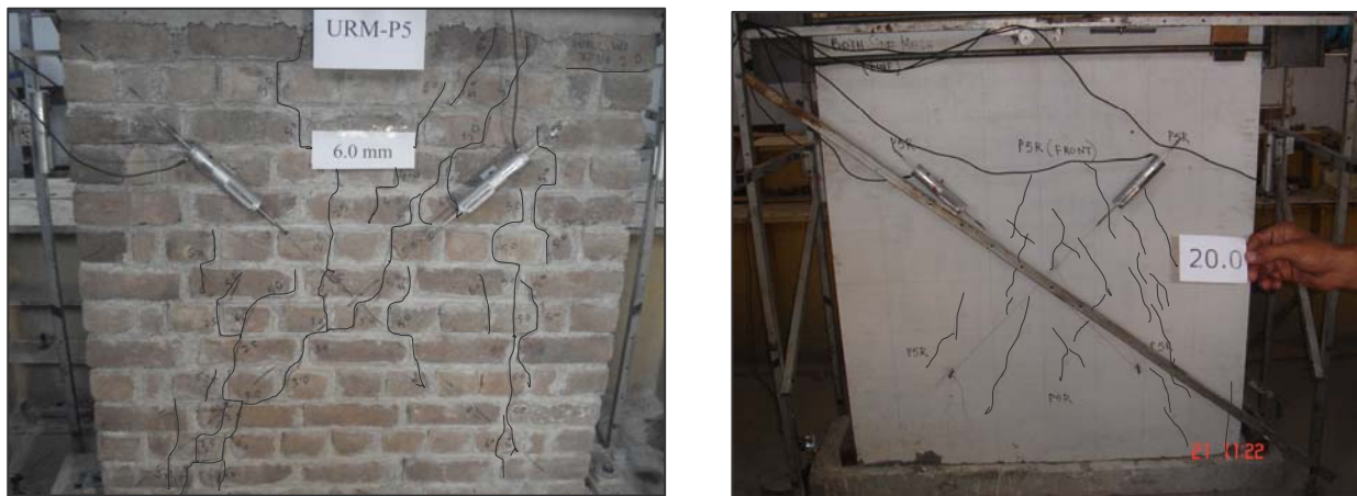
Figure 5. Final damage photograph of specimens P5 (left) and P5R (right)
