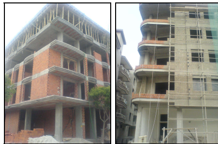
Figure 4. Typical RC building in Turkey. From Izmir, western Turkey.
