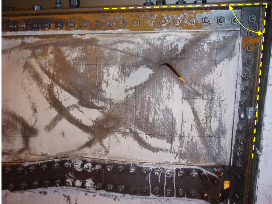
Figure 6. First floor infill plate after the test
