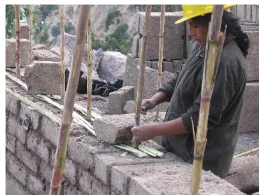
Figure 4 Installation of horizontal reinforcement of crashed canes
