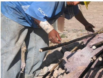
Figure 15 The original method of anchorage Nails are attached to canes to prevent coming off
