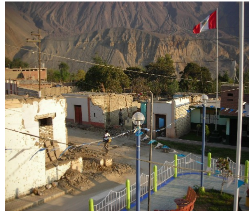
Figure 8 Central area of Zuniga Many adobe houses collapsed
