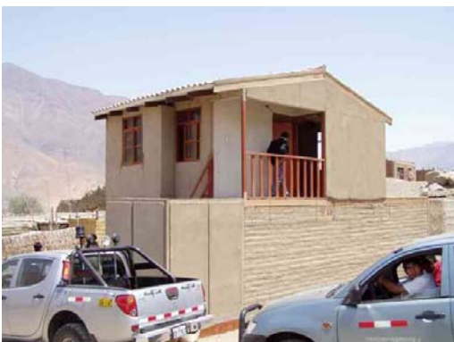
Figure 9 The model house in Zuniga No structural damage
