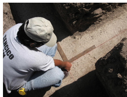
Figure 16 The original method of anchorage Measuring spacing is done precisely
