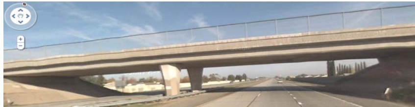
Figure 1. An ordinary bridge with double-column bents and abutments.
