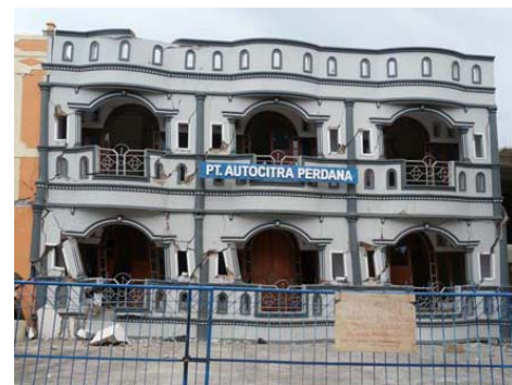
c. Shop houses suffered severe damage after Padang earthquake 2009
