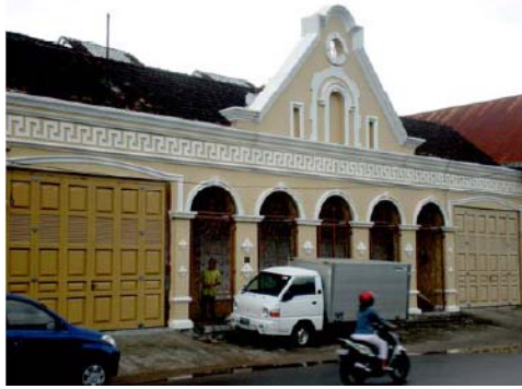
a. Before Padang Earthquake 2009
