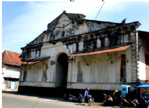
c. Before Padang Earthquake 2009
