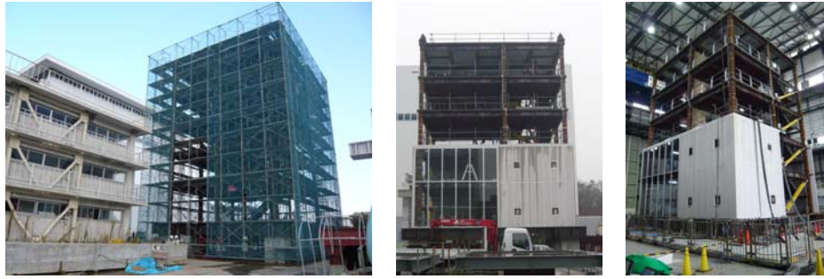
Figure 6. Exterior views of the building specimen under construction (Dec. 2008 and Jan. 2009)
