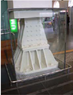
Fig 3. Glass-enclosed riveted joint at Britomart Transport, Auckland Jean Batten State Building in Auckland Central and Hope Gibbons building, Wellington were chosen because of having a complete set of drawings.
