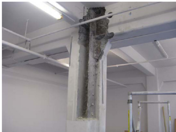
Fig 11. Exposed joint for taking samples
