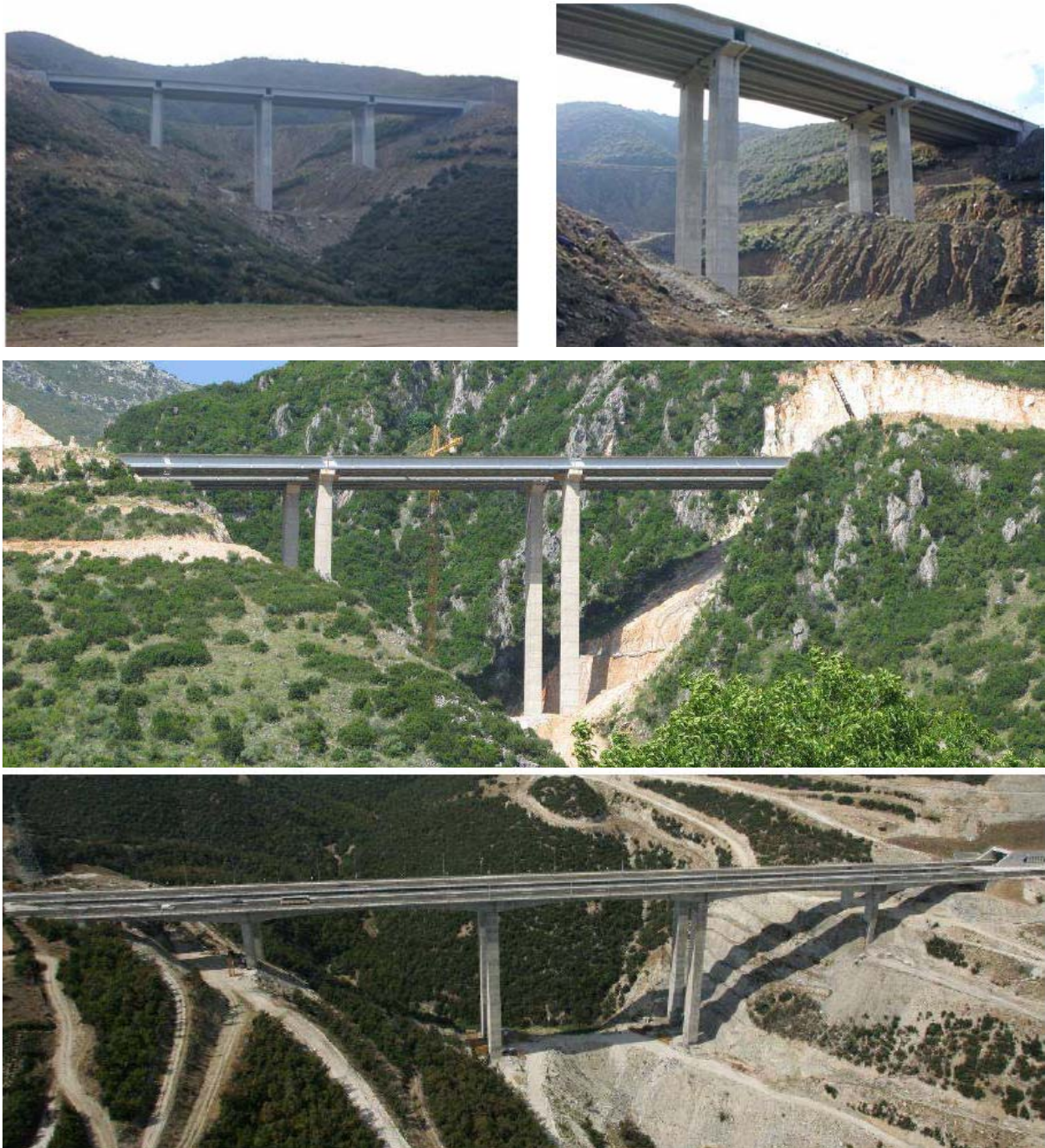
Figure 1. Typical examples of bridges built as twin branches to serve traffic in two directions: (a) 2 nd Kavala Bypass Ravine Bridge studied herein (b) Bridge G4 and (c) Polymylos-Veria Bridge (courtesy of Egnatia Highway S.A., Greece).
