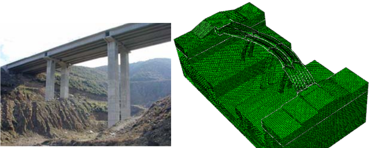
Figure 5. Overview and fundamental mode in the transverse direction of the flexibly supported model of the twin bridge ('3DTwin – 3DSoil', T=1.429\text{sec} ).
