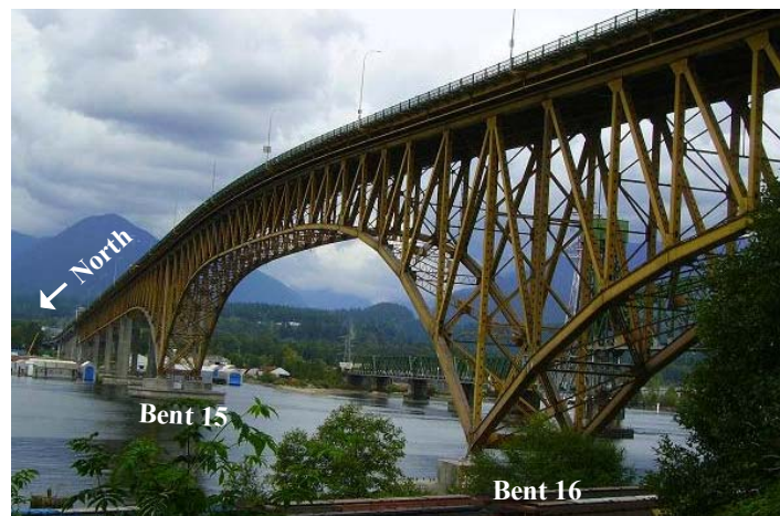
Figure 6. Overview of the IMSNC bridge in Vancouver.
