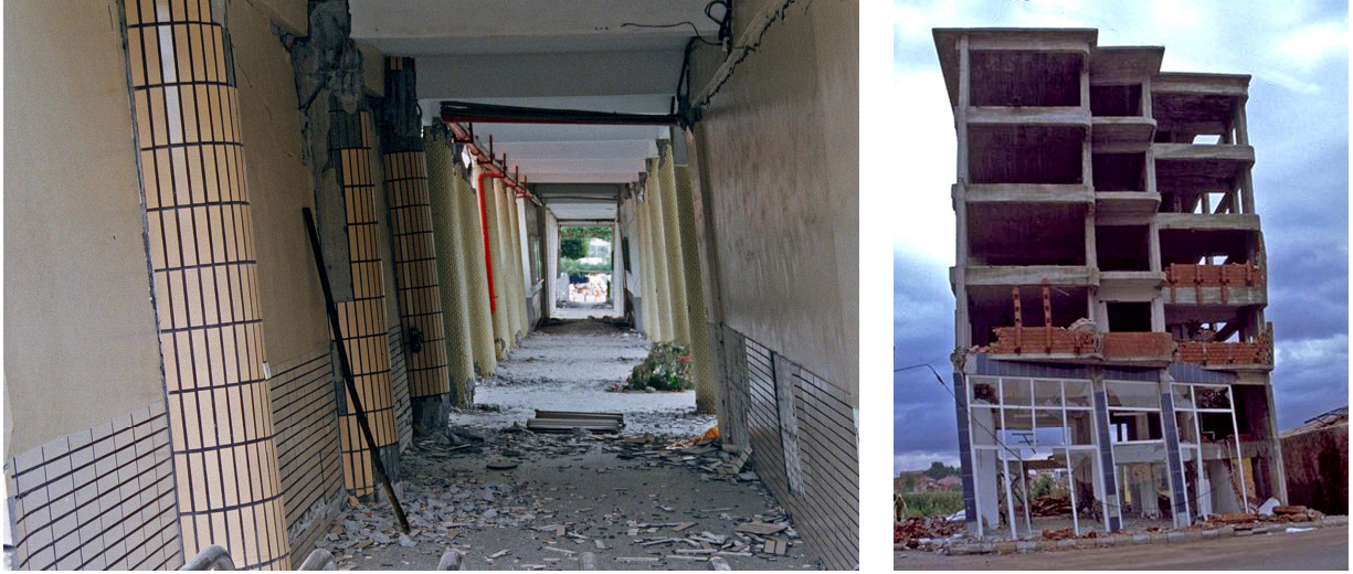
Figure 1. Examples of buildings with residual displacements leading that typically lead to demolition (left photo by M. Bruneau, MCEER; right photo by A. Whittaker, NISEE, EERC, UC Berkeley).
