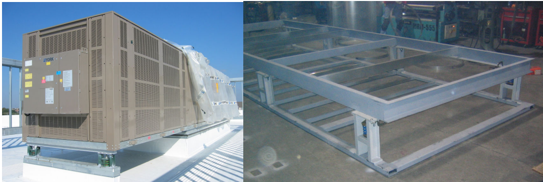
Fig. 8a – A rooftop air handling unit with integral condenser section on isolation curb. Fig. 8b – Internal frames of seismically rated isolation curb.
