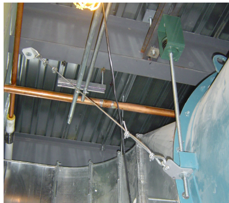
Fig. 6 Isolated and restrained suspended fan
