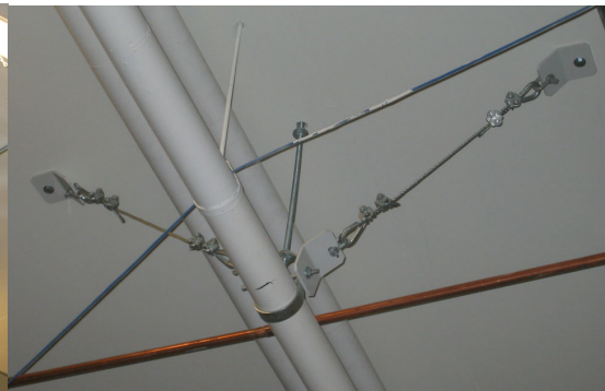
Figure 5b. Cable restraints on a pipe.
