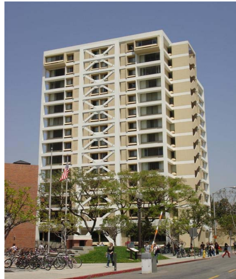
Figure 1(b) Building after retrofit
