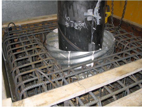
Figure 4. Photograph of Specimen with Grouted Connection Ready for Construction
