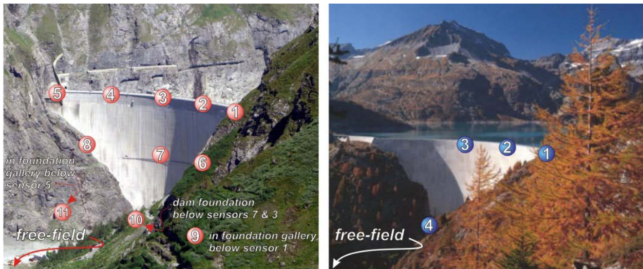
Figure 1: Mauvoisin (left) and Emosson (right) arch dams with approximate strong-motion sensor locations.
