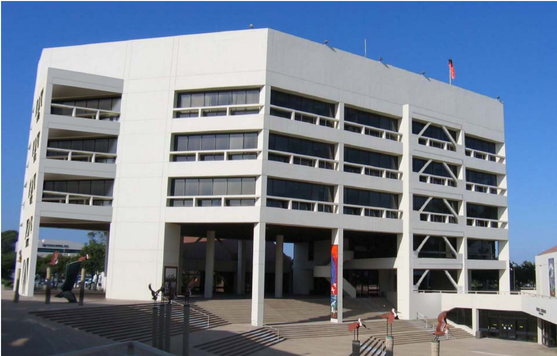
Figure 1. Building after retrofit
