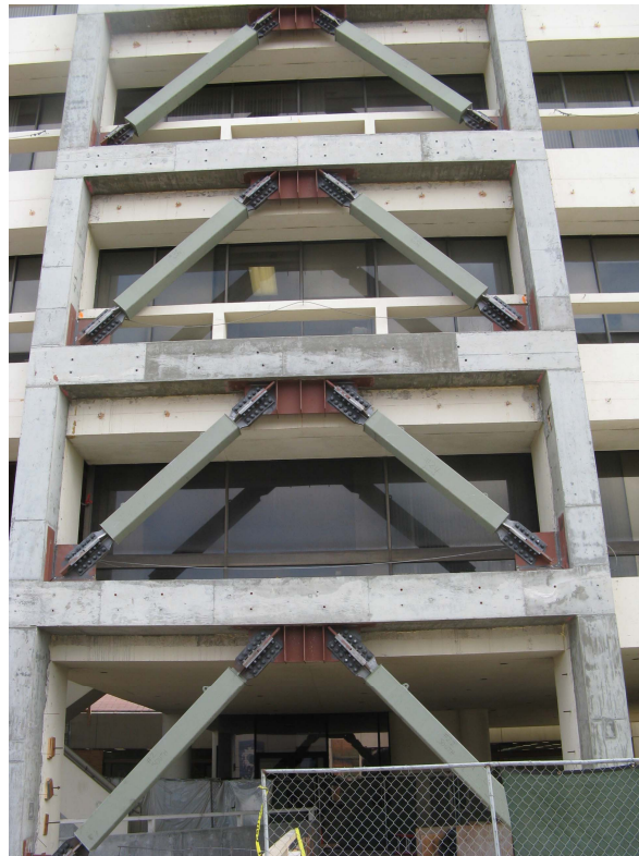
Figure 8. A picture of BRBF members taken during construction
