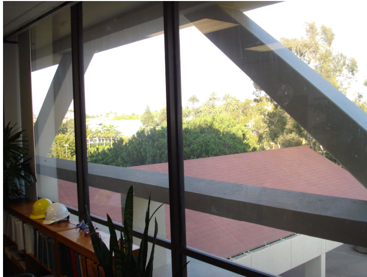
Figure 7. A view of BRBs through an existing window after construction
