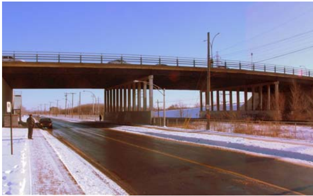
(a) “Emergency-route” bridge
