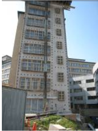
(a) Adding concrete shear walls to Ste-Justine Hospital, Montréal, 2007
