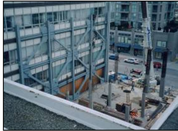
(b) Adding steel bracing to Lions' Gate Hospital, North Vancouver, 2006
