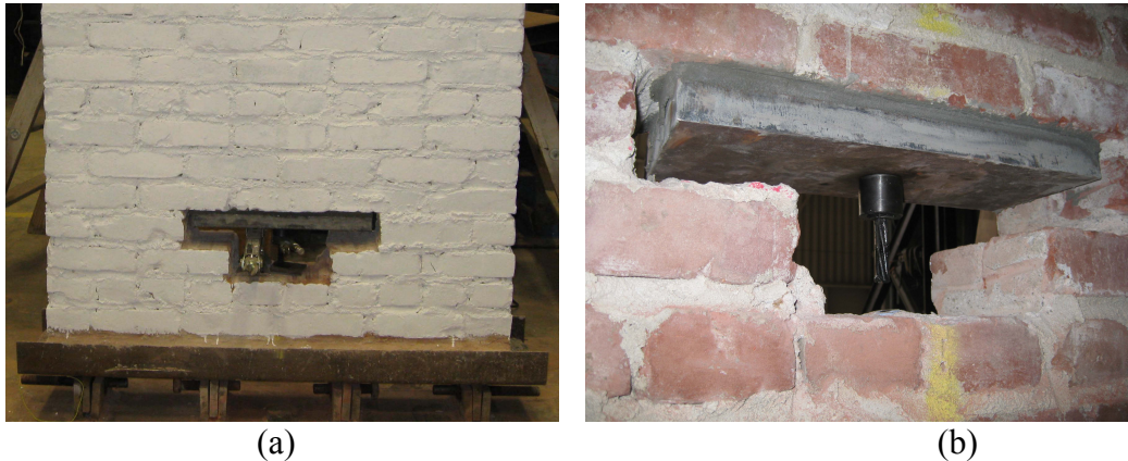
Figure 9: Post Tensioning Anchorage Test (a) Location in Wall, (b) Anchorage Close-up
