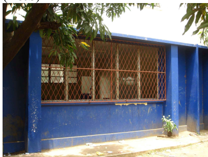
(h) Barred classroom windows of ground floor (S)
