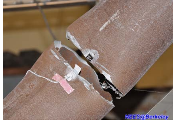
Figure 21. Completely fracture of the brace at first story (West)
