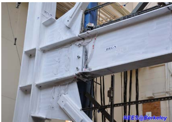
Figure 10. The beam-to-gusset plate splice at east side of lower beam
