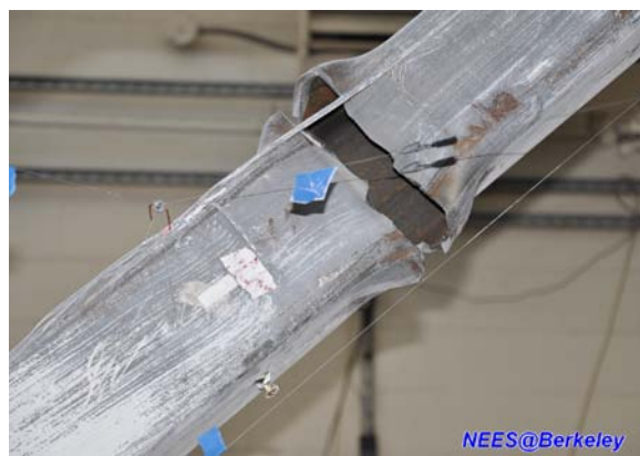
Figure 13. The brace at first story (East)
