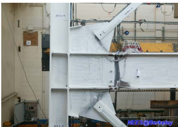
Figure 12. The beam to one-piece gusset plate connection at east side
