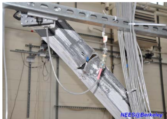
Figure 11. The brace at first story (West)
