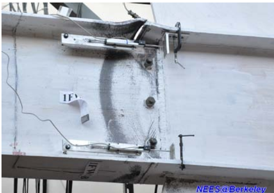
Figure 18. The beam splice at west side
