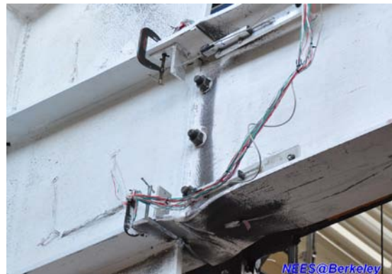
Figure 19. The beam splice at east side
