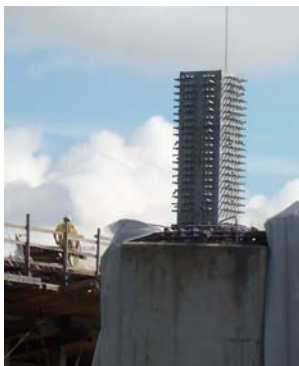
Picture of Pinned Key
