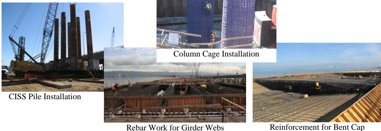
Figure 7 Construction of SFOBB East Span Approach Structure
