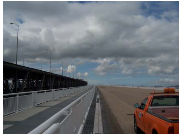
Finished East Bound Deck with Bike Lane
