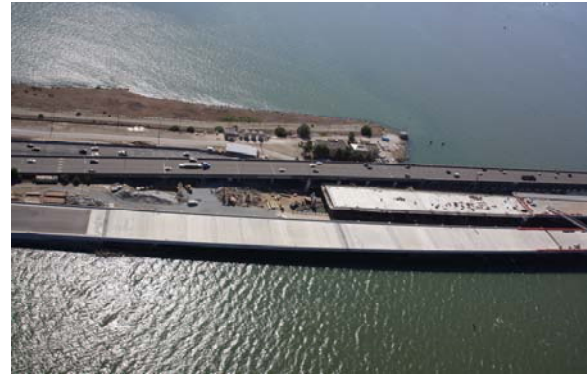
Segment near East Abutment
