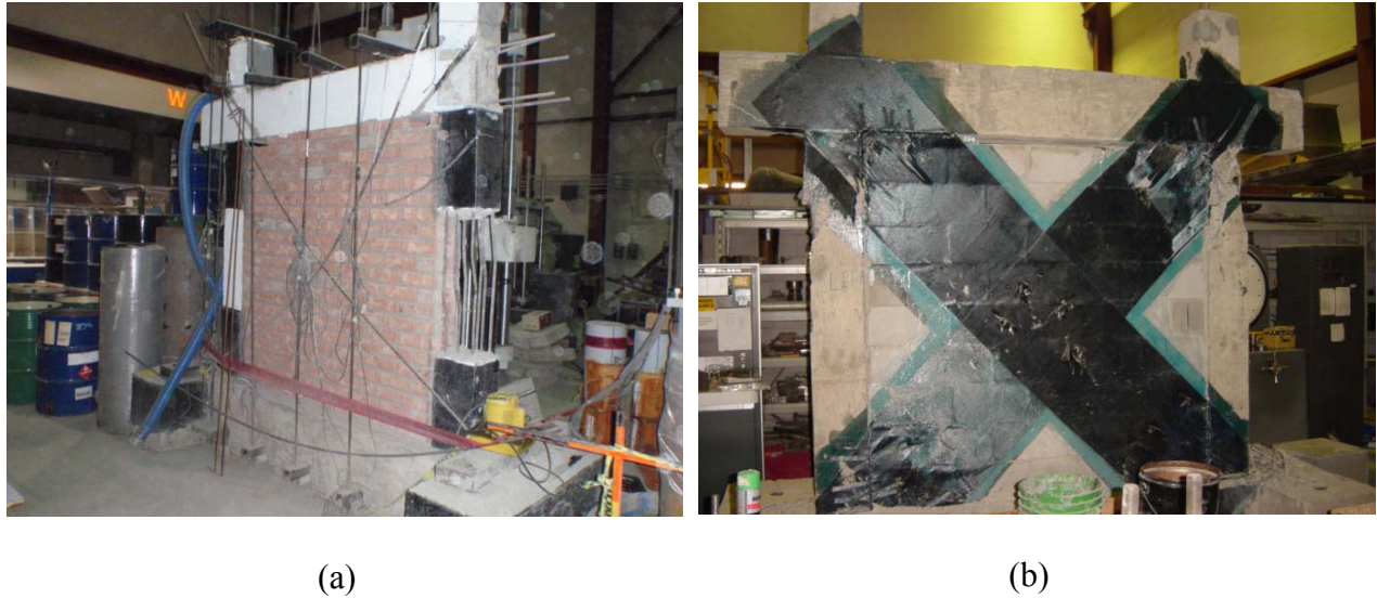
Figure 1. Condition of frames prior repair and retrofitting: a) BR-3; b) BL-3.
