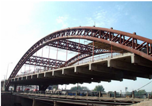
Figure 3. The Beichuan Bridge
