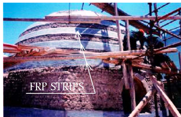
Figure 21. Repair of Al-Aini Dome with FRP
