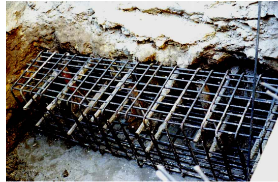
Figure 19. The use of Micro-piles
