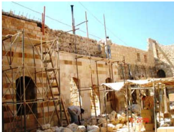
Figure 16. Rebuilding severely damaged walls
