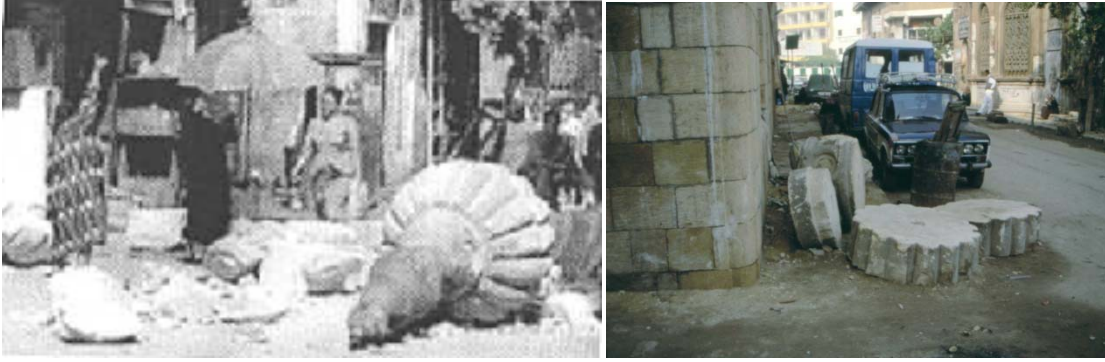
Figure 3. Falling of Al-Ssuity Mosque Bassala During Cairo 1992 earthquake
