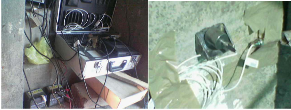
(Data acquisition system)
