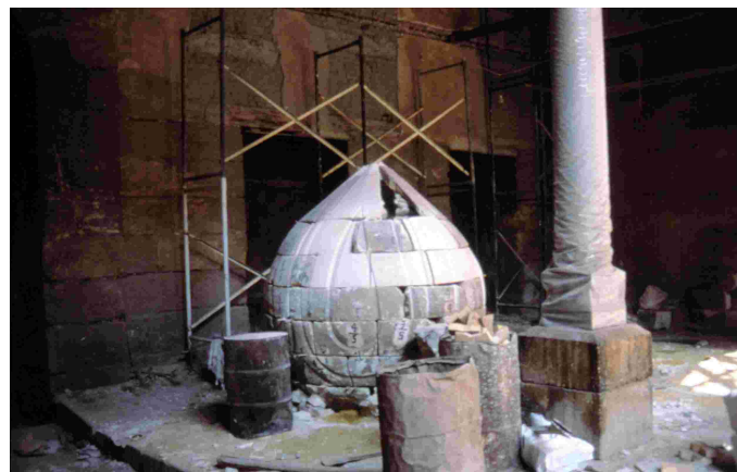
Figure 2. Damage to the top part of North Shaykho Minaret (Bassala) during 1992 Cairo earthquake, with this part reassembled again on the ground during the repair process.
