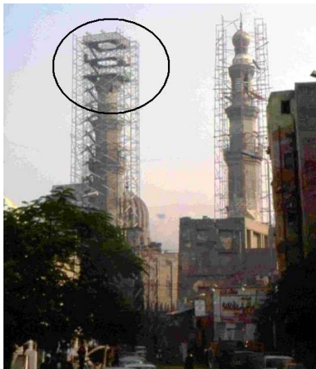
Figure 2. Damage to the top part of North Shaykho Minaret (Bassala) during 1992 Cairo earthquake, with this part reassembled again on the ground during the repair process.
