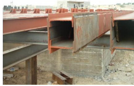
Figure 5. Discontinuity in welding line in cast column
