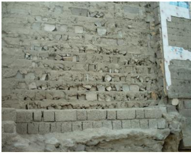
Figure 4. Using material debris to build bearing wall
