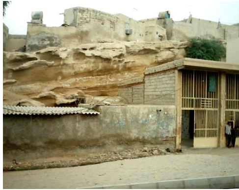
Figure 14. Buildings exposed to landslide
