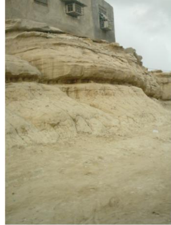
Figure13. The foundation exposed to landslide hazard
