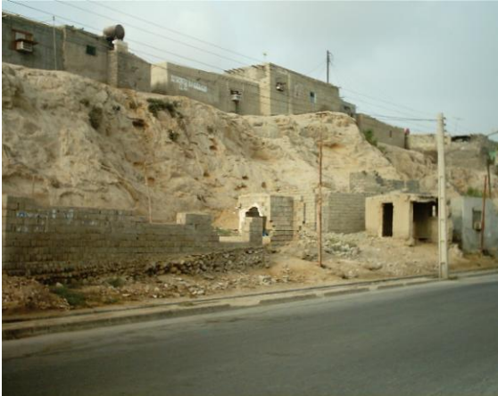
Figure 12. Improper location for construction
