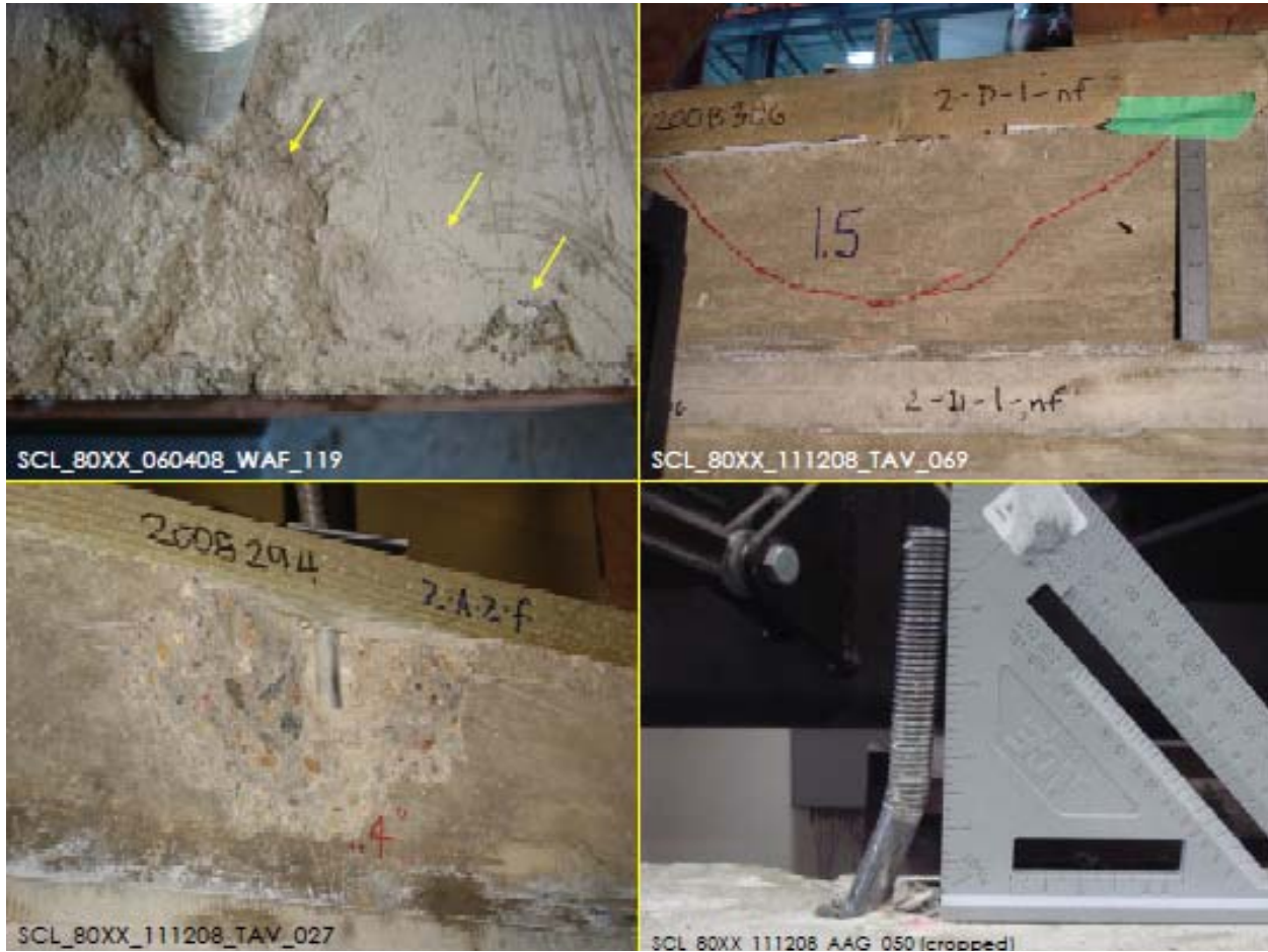
Figure 2 – concrete side break-out development
