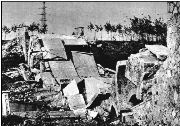
Figure 5. Ye Li Hong Qi Bridge collapsed
