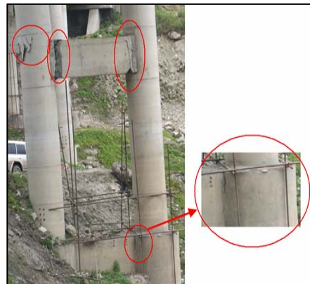
Figure 22. Pier 3# of Baihua Bridge
