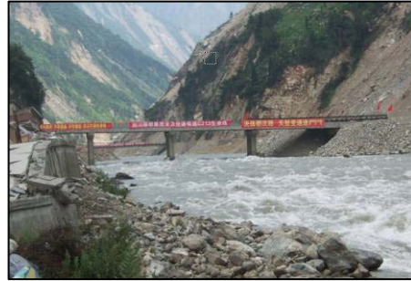
Figure 3. Bridge cross the river
