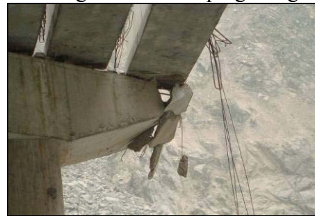
Figure 10. Transverse offset of Yuzixi No.1
