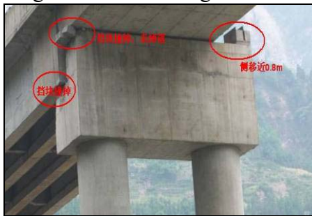
Figure 9. Transverse offset of Baihua bridge
