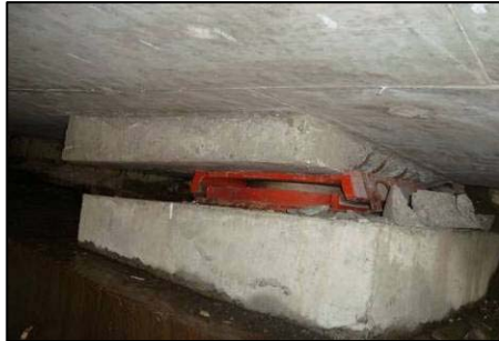
Figure 20. basin rubber bearing
