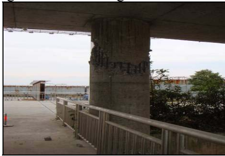
(a) pier inside
