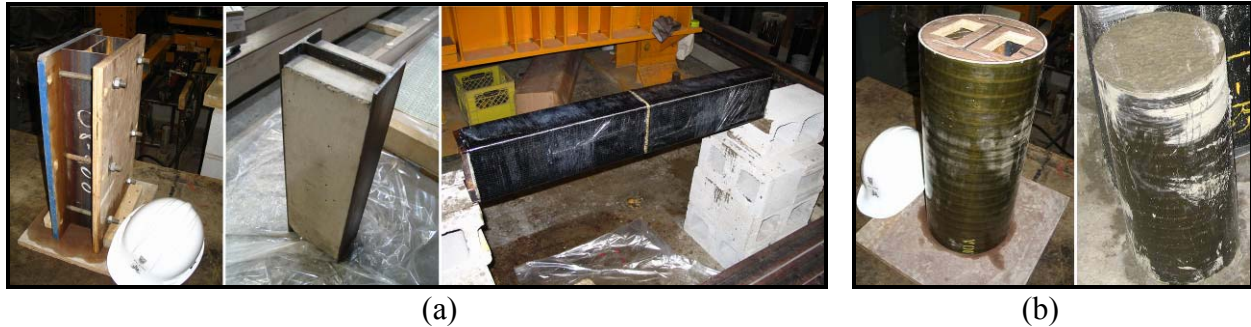
Figure 2. Steps involved in the proposed retrofit procedures utilizing (a) resin impregnated FRP sheets (b) GFRP tube.
